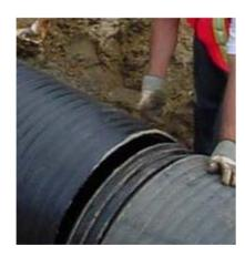
Step 2: Place pipes in straight alignment
