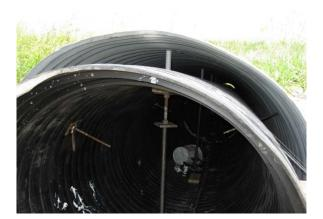
Using jacks to hold the pipe down.
