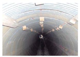
A side rail wooden blocking to assist with the minor bends.
