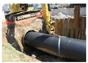
Different ways to inserting Weholite liner into the host pipe.
