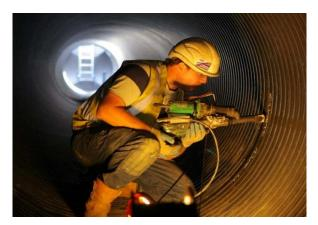
The inner wall (IW) weld.
